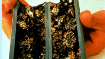
Zebra mussels in a cut-away pipe
